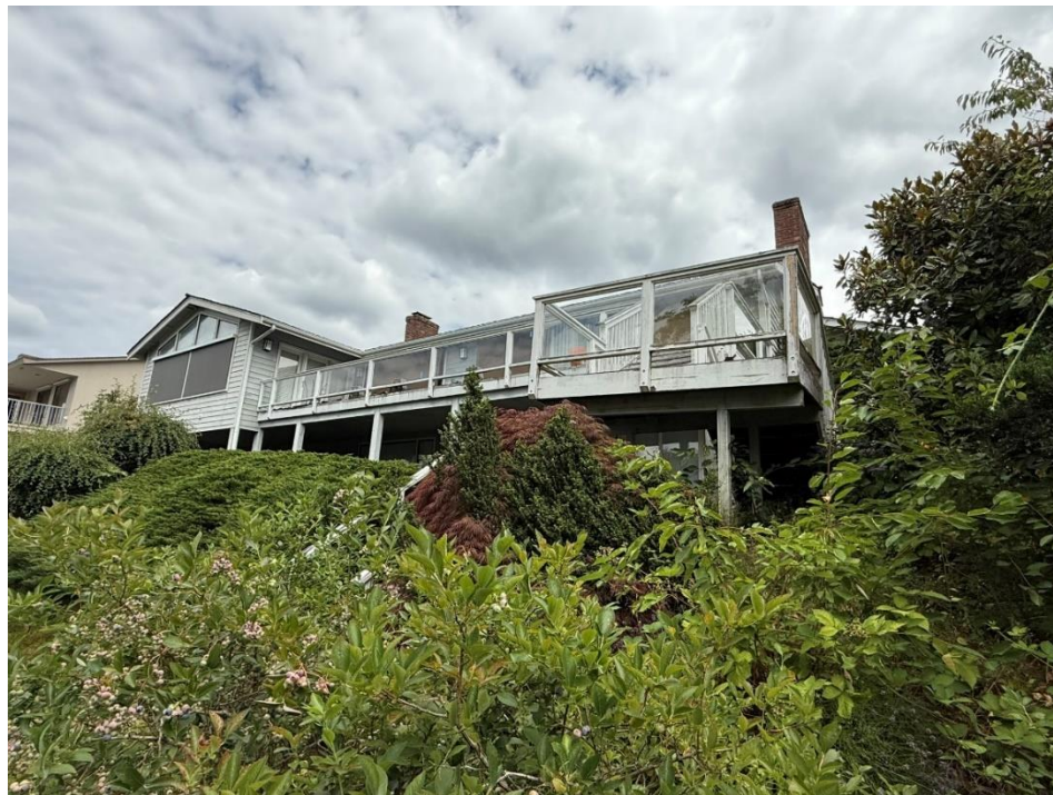
Plate 1. Existing house and proposed deck location, looking northeast (7/14/2025).
